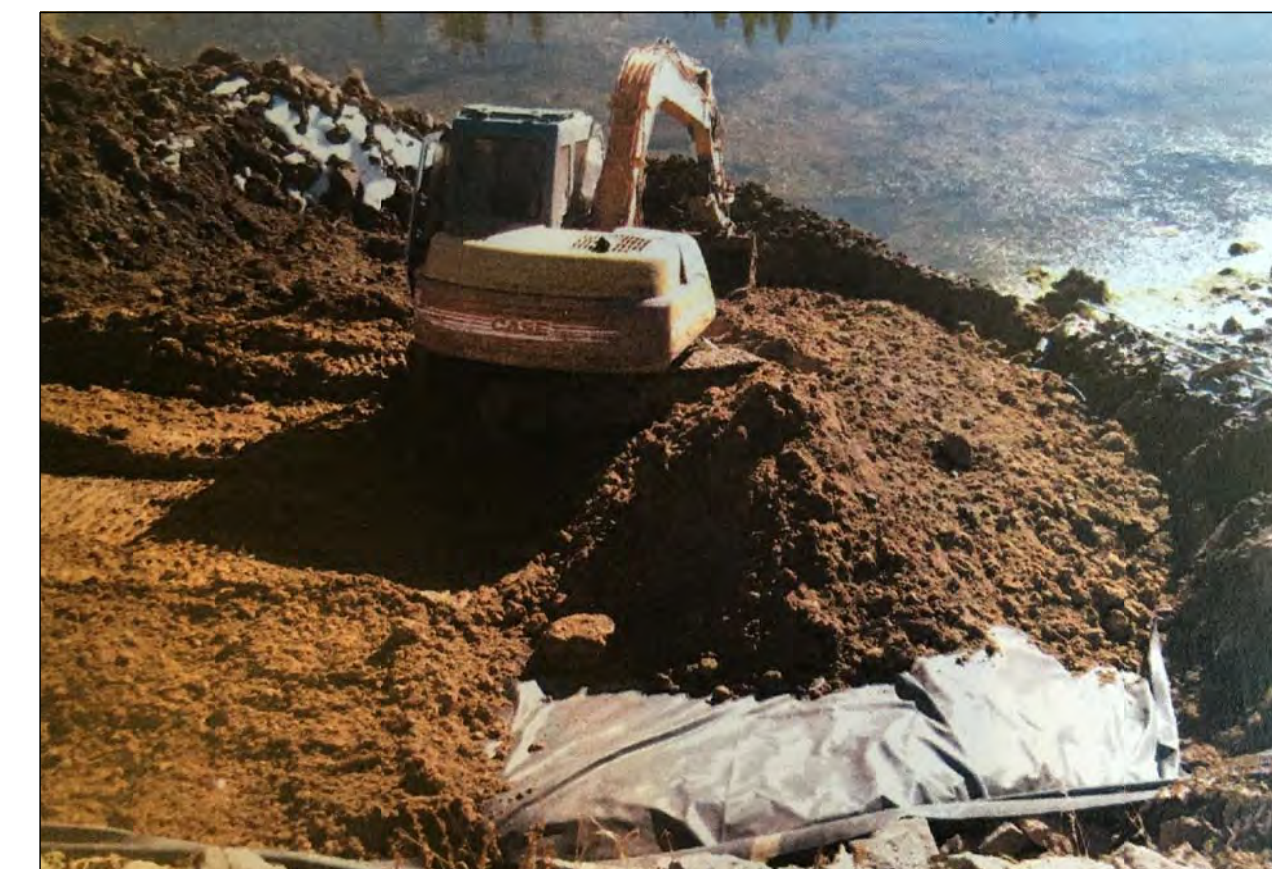
STEP 4: Place 12-inches of backfill over liner and compact.
