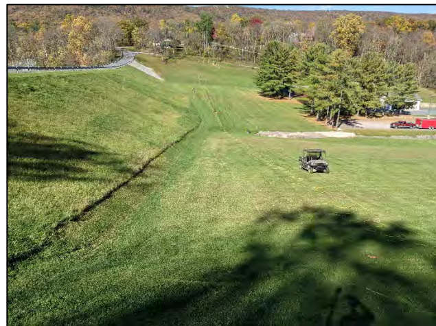
Figure 2. ERI Field Investigation
