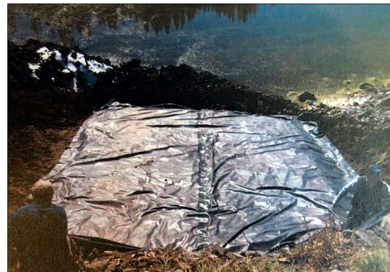
STEP 3: Install 45-mil EPDM Liner.
