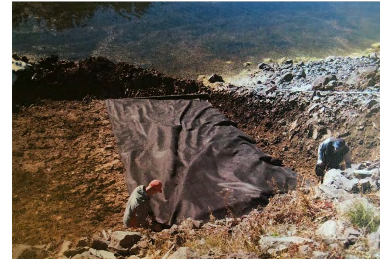
STEP 2: Install 8 oz. Mirafi 140N (or approved equal) Filter Fabric.
