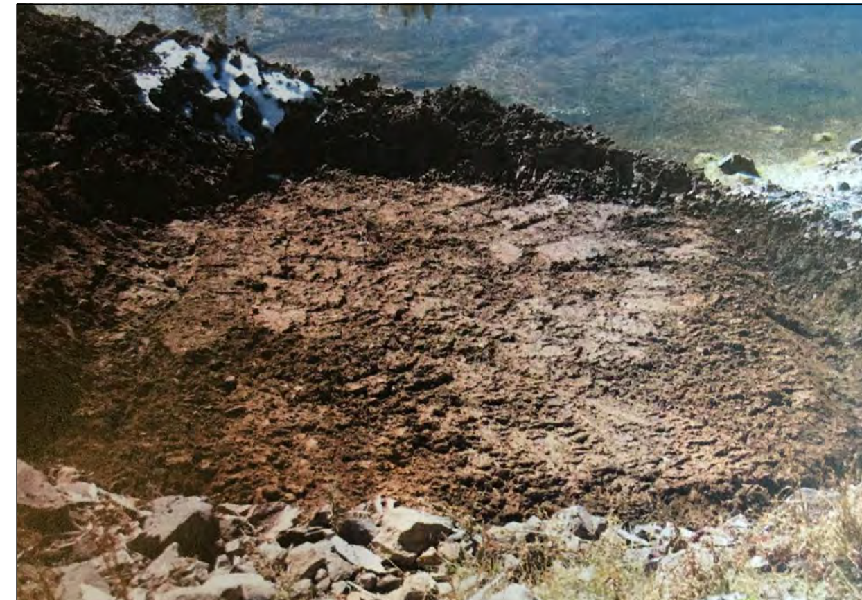
STEP 1: Clear & Grub Upstream Slope of Embankment in proposed Liner Area, Expose Existing Liner Anchor Trench, Compact, and Prepare Subgrade for New Liner System. Dig remaining anchor trenches.
