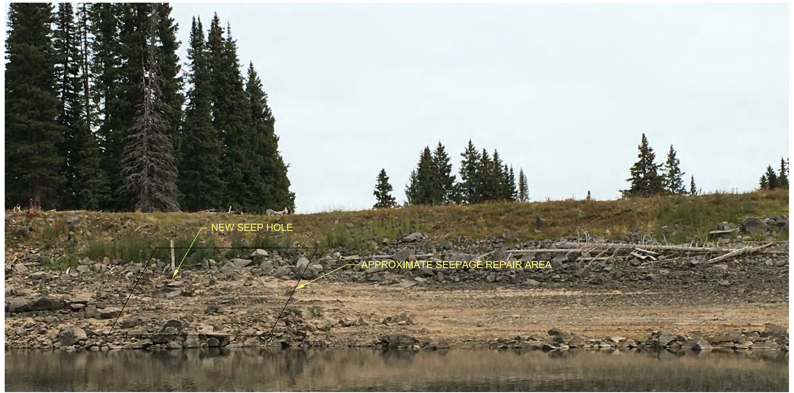
POND AND UPSTREAM DAM FACE
